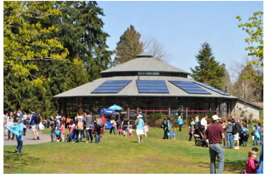
Solar panels on a park pavilion. Image Source: Solaripedia
